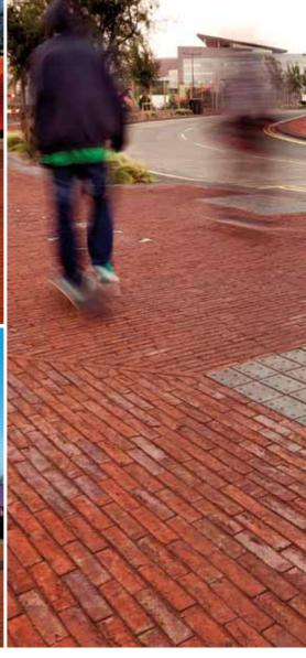
the Porth Teigr area, durability was also one of the priority criteria for the design team and Cardiff City Council. Due to the inherent performance capability of fired clay products, the Slimpave Koln Red is a hard-wearing paver and therefore ideal for the job.
