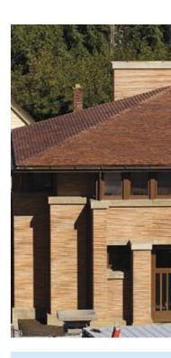
In the brown flamed clay roof tile from French roof tile factory Pontigny Aléonard, a tile was found that matched the original weathered roof tiles.
