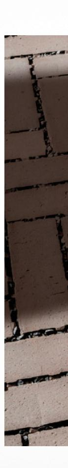
Because the water flows away from the clay paver faster via the wider joints, it also decreases the risk of growth of algae, moss and weeds in the joints. This is extra beneficial for the appearance and ease of maintenance of the pavement.
