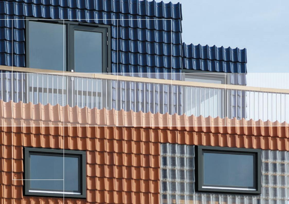
oramic clay roof tiles have been successfully used in apartment block construction. The evidence can be found in the growing numbers of projects in which clay roof tiles are used as a maintenance-friendly wall cladding material. It is the ideal material to accentuate an unusual architectural design, to give different parts of a building a distinctive appearance, or to add a feeling of unity to a project.
