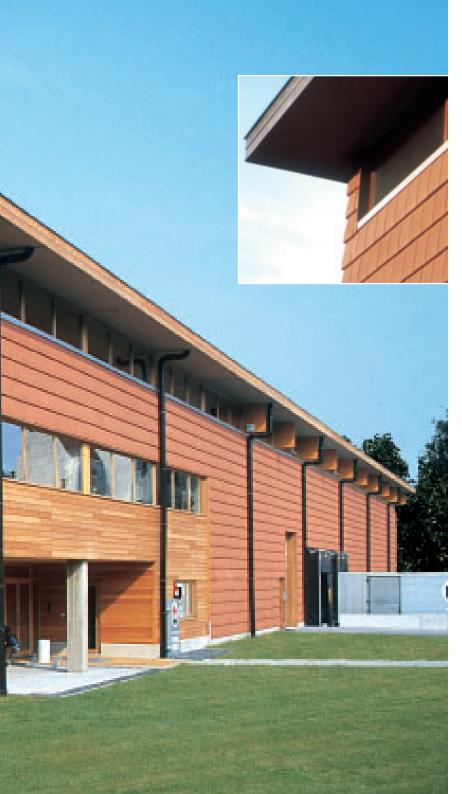
The use of clay roof tiles as wall cladding is remarkable and trendsetting.
