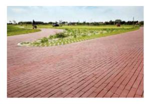
The new UrbanA+ paver, which was specifically developed for pedestrian zones and squares, was used for the footpaths. The pressed clay paver, fired especially hard, is also available in black and violet.
