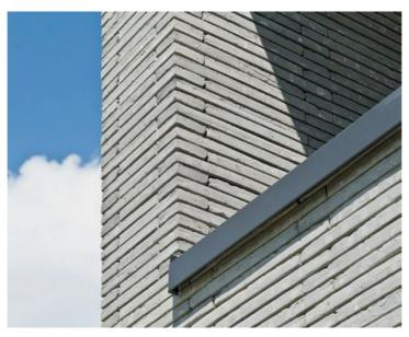
exterior blinds. Proportions and details are accurately coordinated with the light grey façade and the cubic standard shapes. The special laying of the bricks and the play of light and shadows resulting from the deliberately omitted jointing clearly visualise that every water-struck brick is a unique specimen. The result is a fascinating façade structure.
